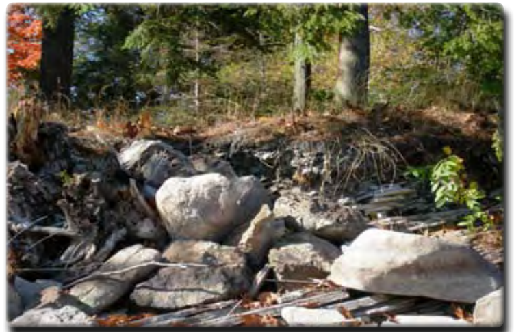
Erosion on the shore of Big Rideau Lake Photo: J. Trant
