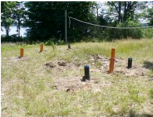
6 inch mortars buried in the volleyball court for the really big display fireworks. They are yet to be loaded, armed and connected to the control panel.
